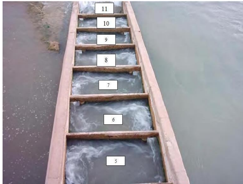
Figure 2. Fishway at Karkheh Hamidieh Diversion Dam in Iran (Filli et al. , 2007)
